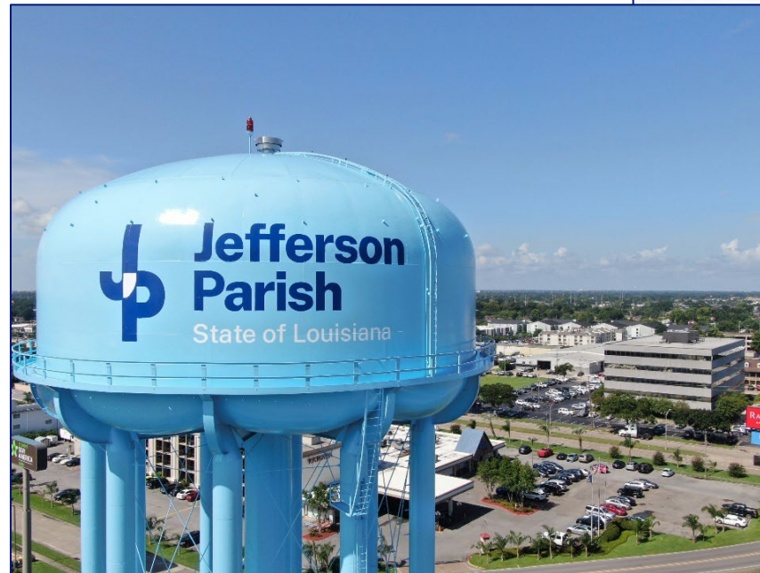
I-10 / Causeway Blvd. Water Tower
