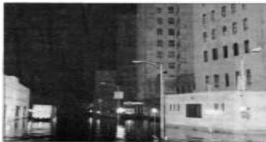
FLOODING Floodwater surrounds Charity Hospital, just days after Hurricane Katrina inundated the city. Basement flooding wrecked wiring and plumbing and trashed medical equipment, much of which was so old that replacement parts aren't made anymore. STAFF PHOTO BY ALEX BERGSON
